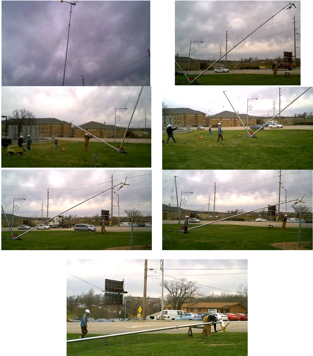
Figure 1: 1.2kW Bergey Wind turbine is brought down to earth in 2 minutes. This can be viewed on http://www.youtube.com/watch?v=sXntmY7B_f4
